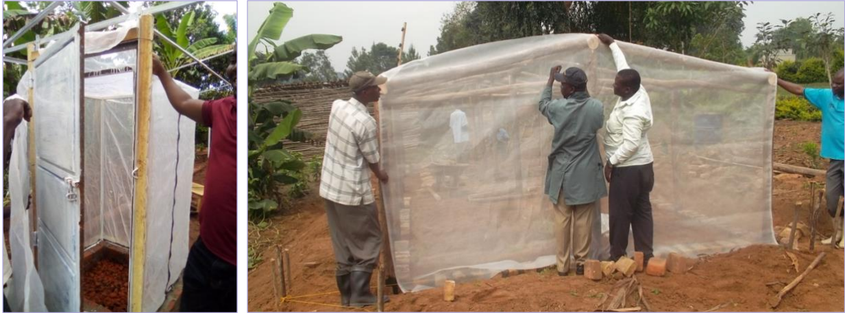
Plate 5: Fitting the sewn net on the wooden frame (Credit: Sam Namanda)
