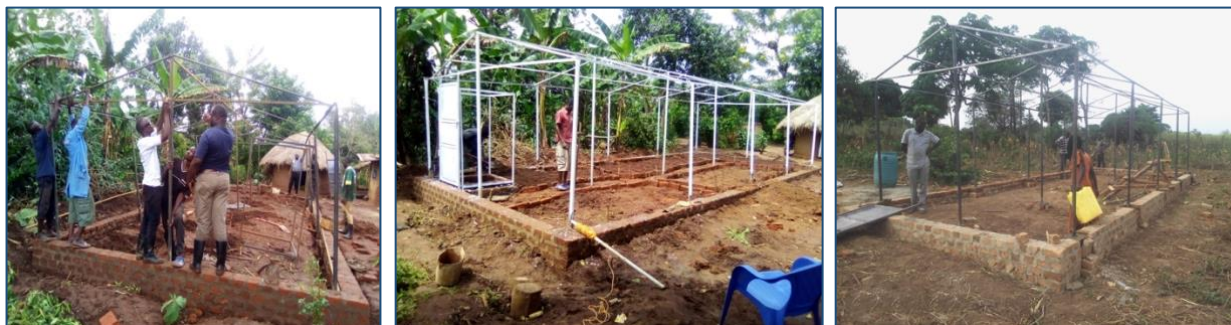
Plate 2a-c: Construction of foundation and house frame (Credit. Sam Namanda)
